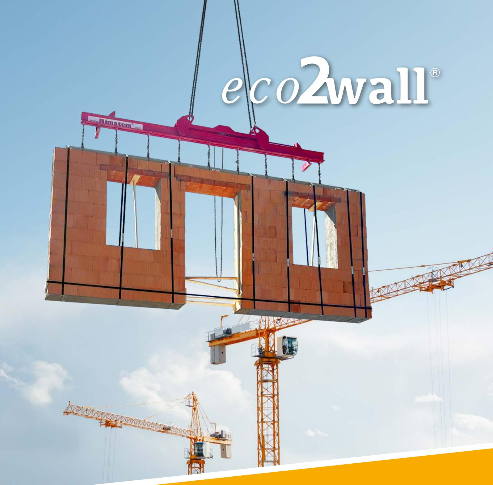
A large-scale construction site under a clear blue sky with scattered white clouds. In the foreground, a large, rectangular brick wall element is being hoisted into the air. The element is made of reddish-brown bricks and has three rectangular openings. It is suspended by a red metal crane beam with the 'Rimacem' logo. Black straps are used to secure the element. In the background, several yellow tower cranes are visible, along with the skeletal structure of a building under construction.
